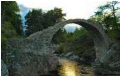
The Queens Bridge in Scotland picture taken from www.armin-grewe.com/holiday/scotland2005summer/queens-view.htm
